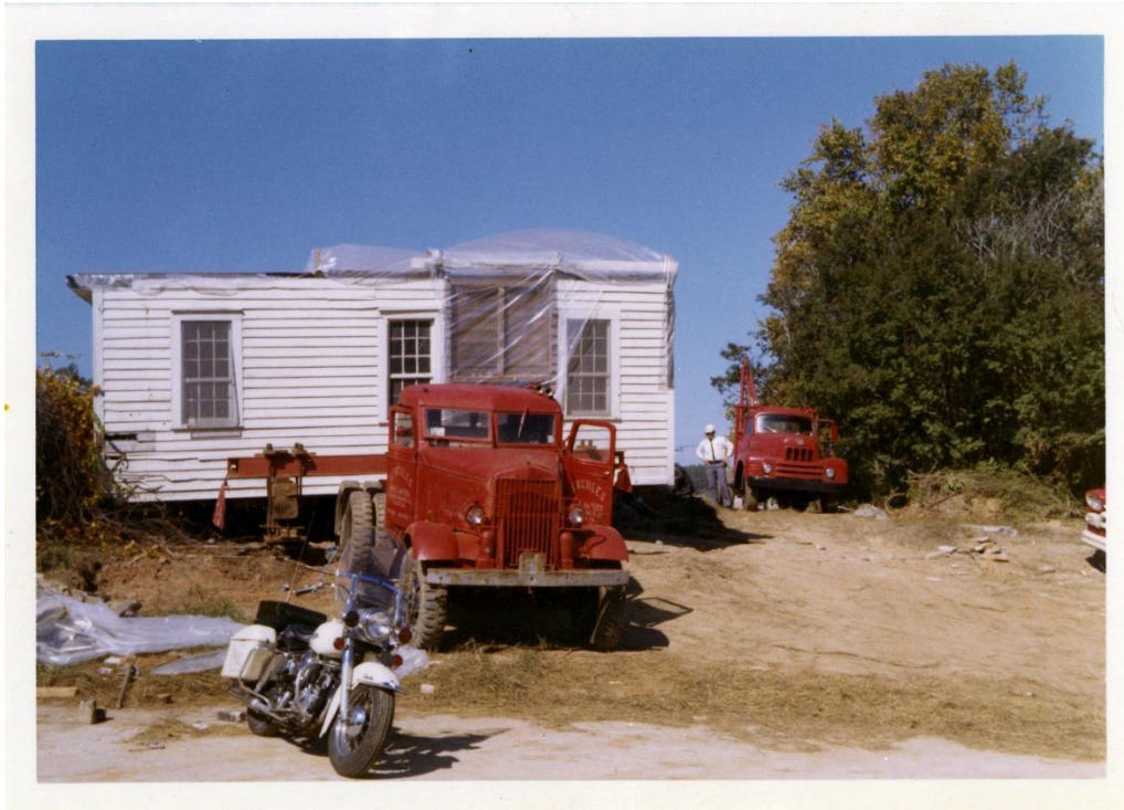
Moving ca. 1845 Tullie Smith House to Atlanta Historical Society, 1969. The upper floor of the house was completely disassembled, while the lower floor was moved largely intact.
