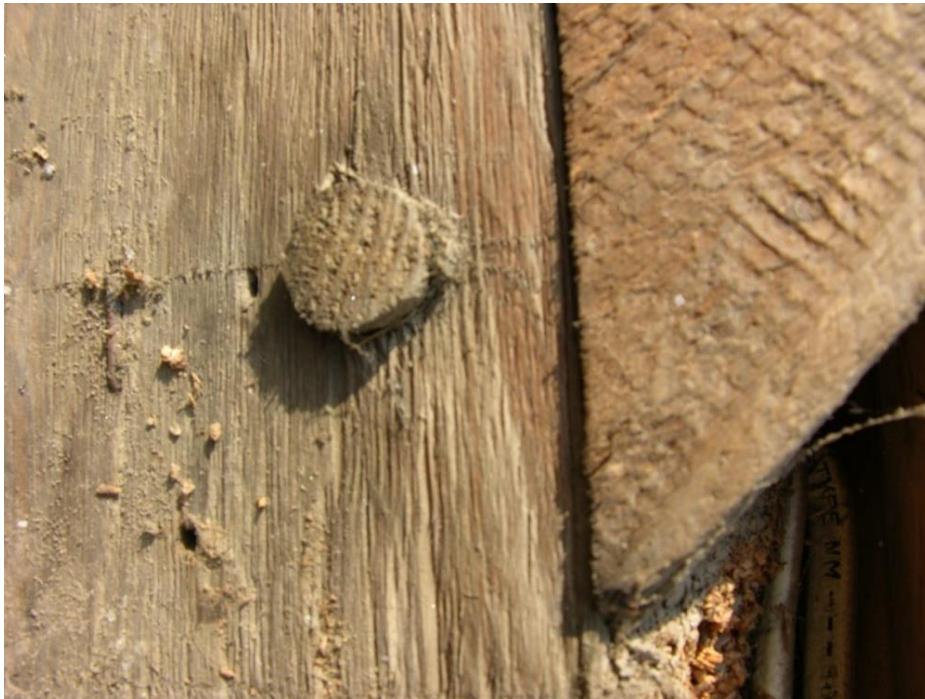
Close-up view of peg used in framing of Tullie Smith House
