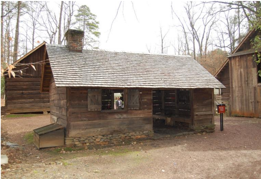
Reconstructed blacksmith shop at Smith Farm Atlanta History Center, present day.
