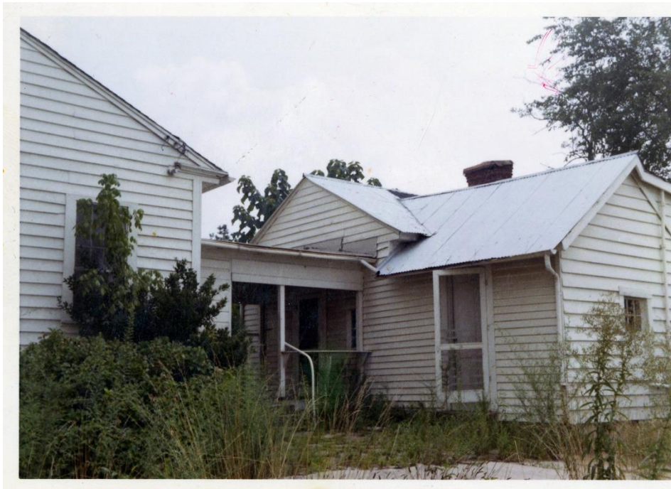
Close-up view of detached kitchen on its original site on N. Druid Hills Road before house and kitchen were moved to the Atlanta Historical Society, 1969. Note breezeway that by then connected the house and the kitchen.
