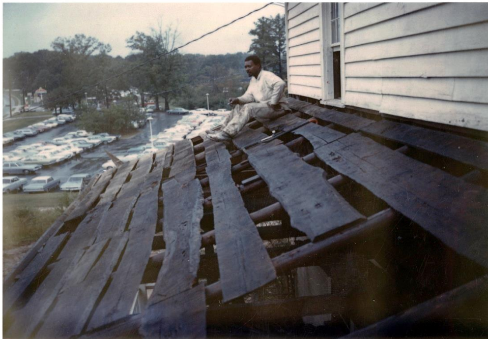
Disassembly of ca. 1845 Tullie Smith House for move to Atlanta Historical Society, 1969. This is the shed roof covering the two rear first floor rooms. Note encroachment of modern development in background.
